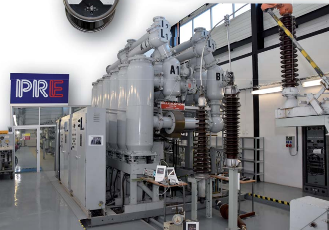
Original 110 kV switchgear dating back to 1980 (Delle Alstom)
